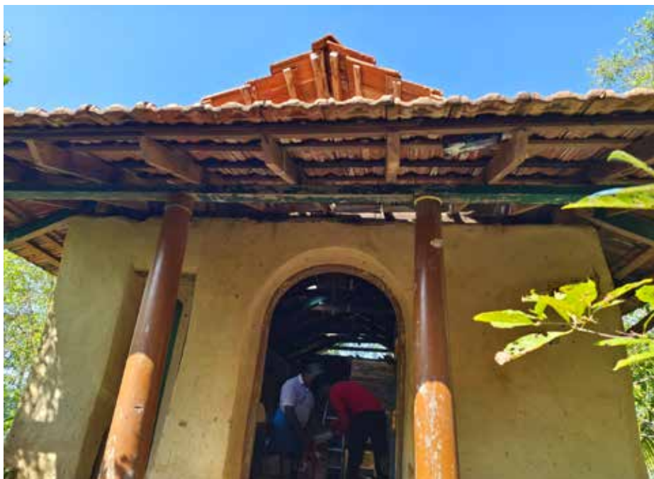
Mudhouse about 250 sq ft, rosewood pillars, Thinnai, roof made of used tiles
